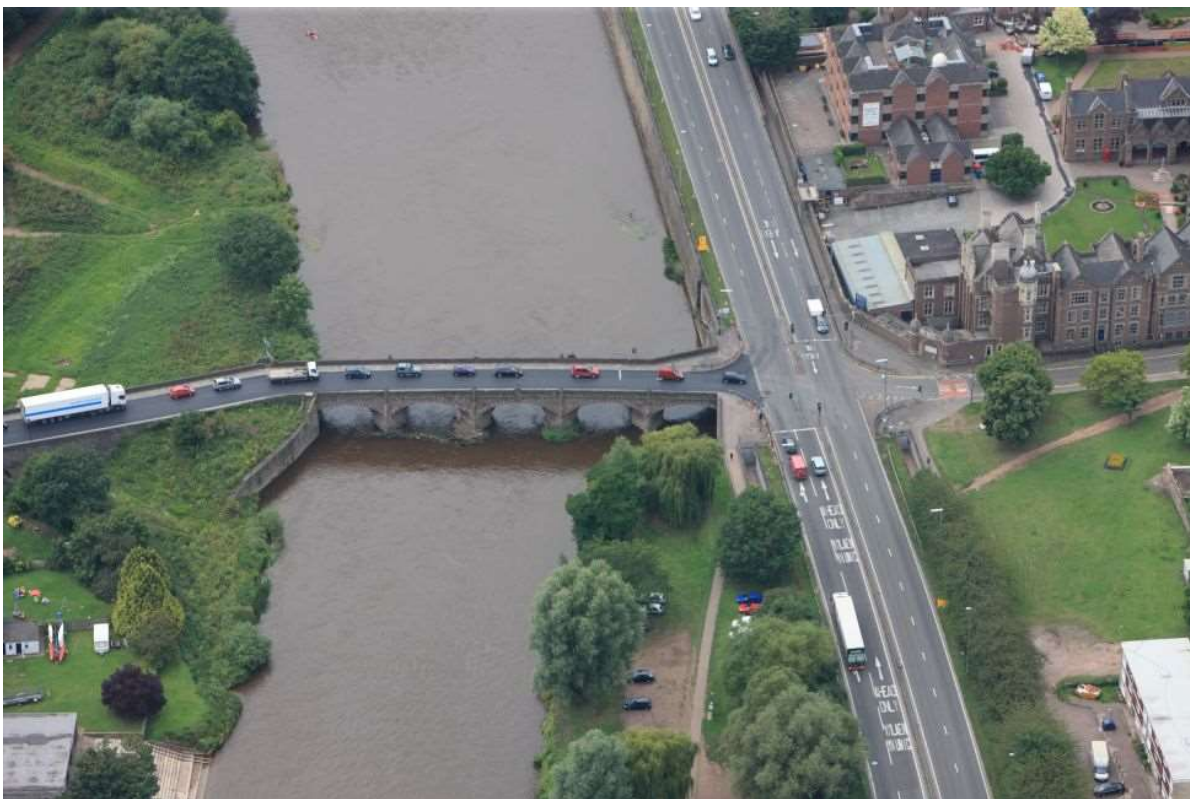
Plate 6 – View of the Grade II listed five span arch masonry Wye bridge
